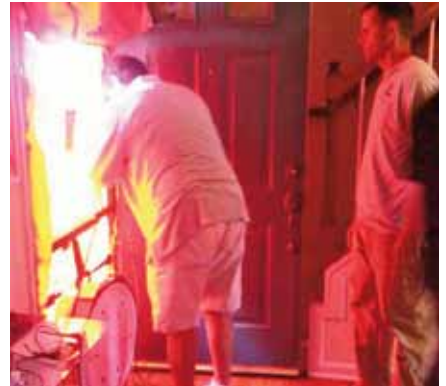
CHEC lineman Richard Augustson and BPI classmate set up the blower door test during residential energy auditor training.
